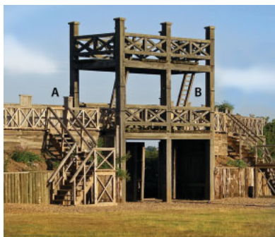
Replica of Roman ladders: (A) attic ladder, resembling a staircase (B) dovecote ladder
